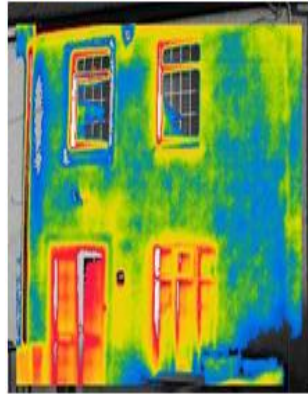
Front Elevation After Pumping
