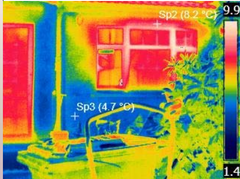
Hollow block extension
